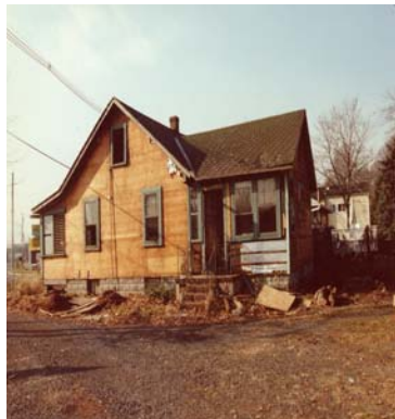
BEFORE: 1235 Rt 1, Edison NJ
